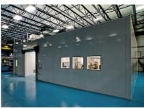
The cleanroom is certified to the ISO 14644-1 Class 8 standard. The 2000-sq-ft facility houses six electric injection molding machines from Toshiba Machine's EC Servo Electric Series outfitted with high-pressure water controllers to allow more versatility in resin selection. The cleanroom also features removable panels to accommodate future expansion.
